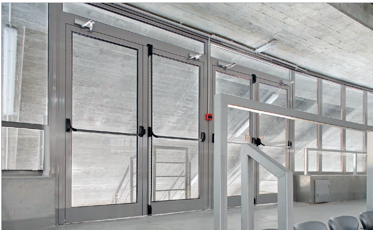
Sports Hall, Zadar, Croatia (Photo: Robert Les)
